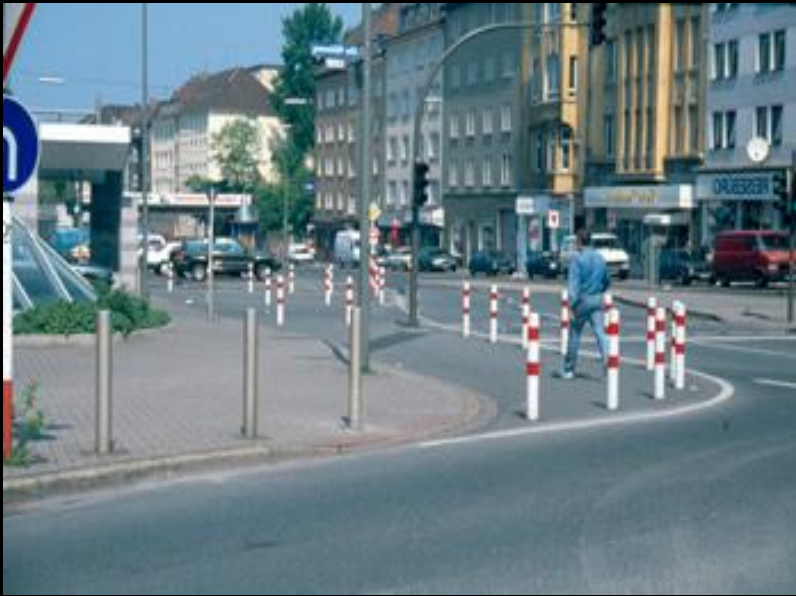
Piloting a curb extension
