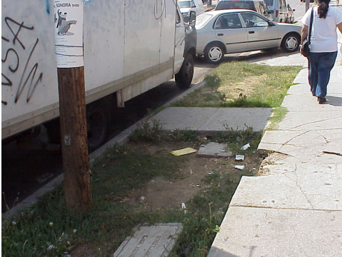
Narrow and broken sidewalks make walking a challenge
