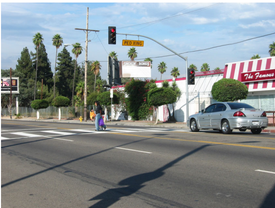
Example of a pedestrian-activated crossing signal in Highland Park
