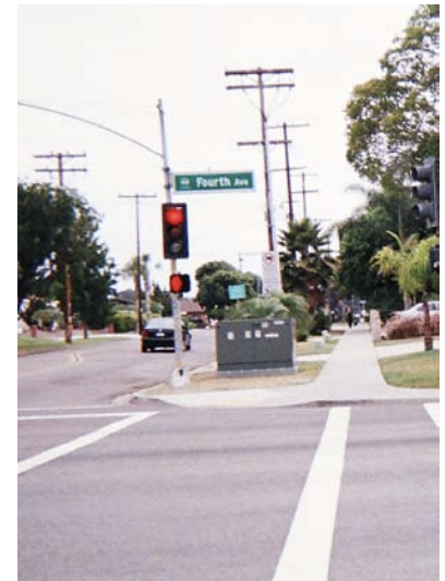
A Photovoice photo indicating that there are no push buttons to activate the walk signal
