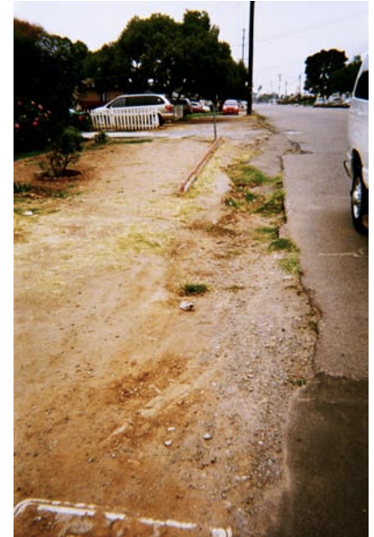
A Photovoice photo reveals missing sidewalks that are difficult to navigate for seniors and impassable for the disabled
